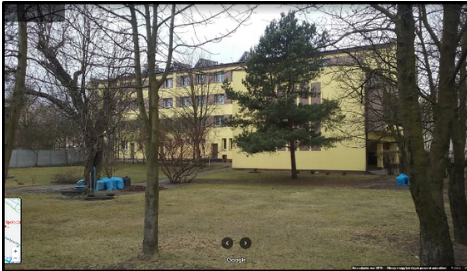
Photo 27. A side view of the DPS building
